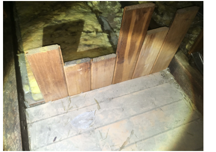
close-up of wall/ceiling joists
